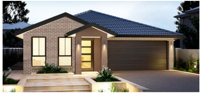
NEW TRADITIONAL MASONRY
